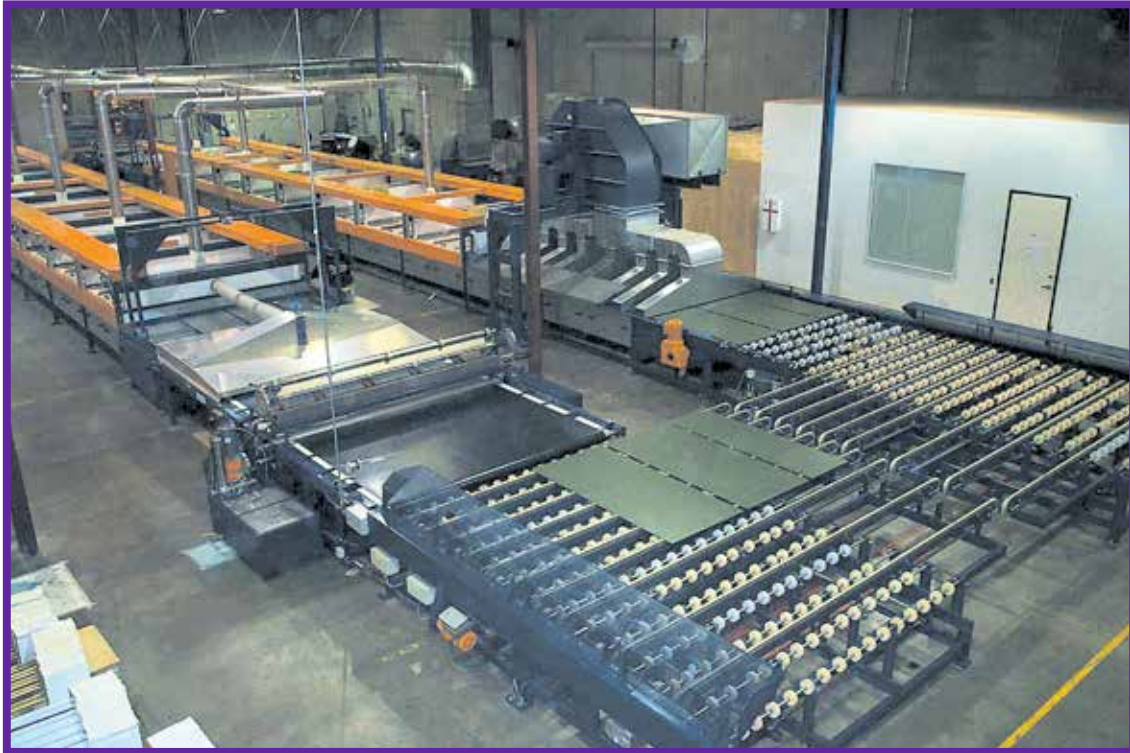
Contractors Wardrobe ® 's Klöpper Mirror Conveyor - located in Sacramento, California. The efficiencies of the line along with the "Copper-Free" chemical solution are environmentally friendly and improves the quality and life of the mirror.
